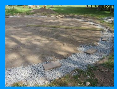
Backfill with crushed stone around the pavers that will be a base for wall uprights. Lots of trips to the stone pile with the wheel barrow and more shoveling to unload.
