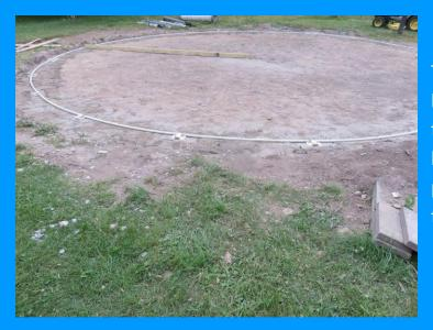
The center was now ready for basic raking and landscape fabric. After the fabric, we hauled sand to the center and put up the walls. How can 30 foot diameter look so small?
