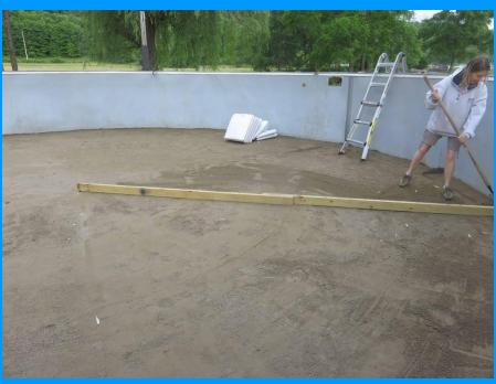
Once the sand was leveled and tamped in place, the gorilla pad was installed. \$200.
